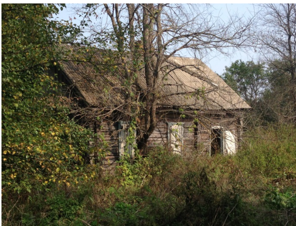
There were many abandoned houses at severely contaminated areas
